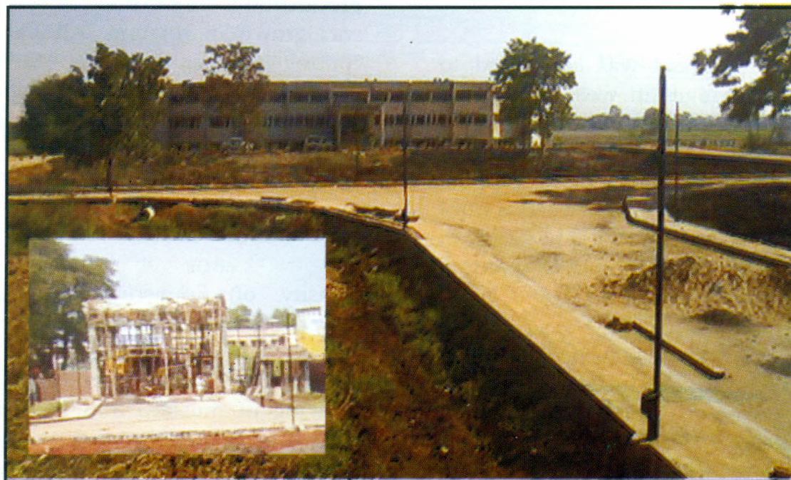
Fig.-2: Construction of approach road and gate of the centre
